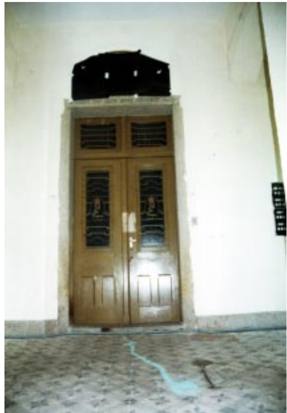
Art deco door - a 20th-century alteration
