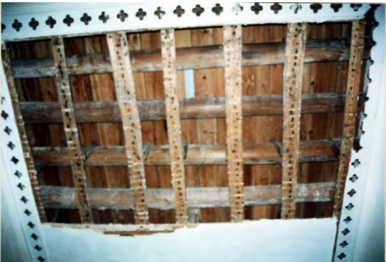
Original floorframe over the central corridor of the 'nave'
